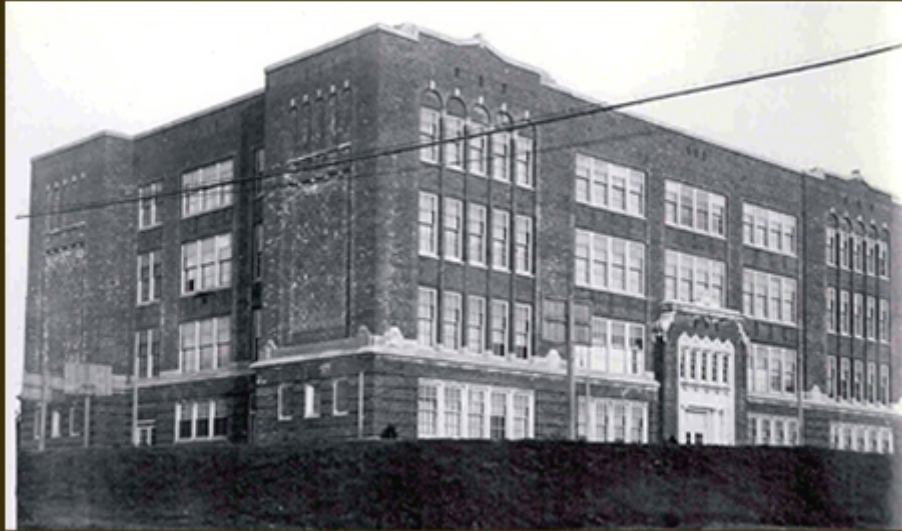
Northeast Junior High - Front Facade Historic Photo
