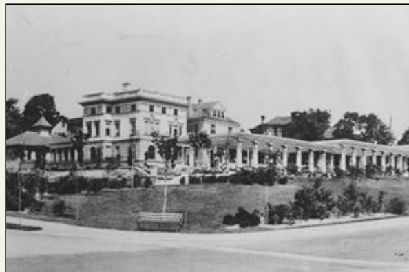
Looking northwest from the southeast corner of 11th and Paseo.
